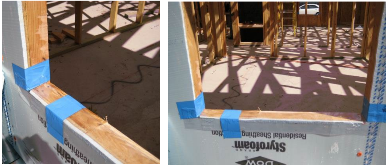
Figure 6-11. Window Sill Pan Installation
