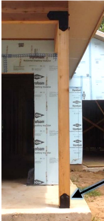
Figure 4-37. Installed 6x6 Porch Post
