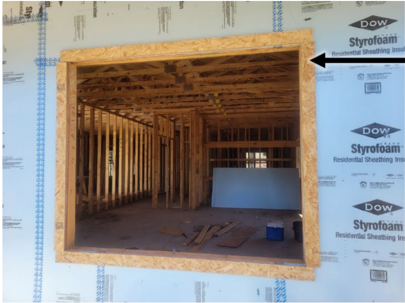
Figure 6-17. Window Furr Out for Brick
