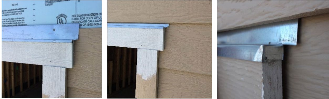
Figure 9-37. Z-Flashing Over Garage Trim
