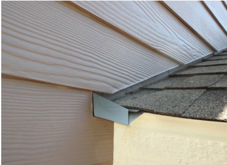
Figure 10-12. Installed Diverter
