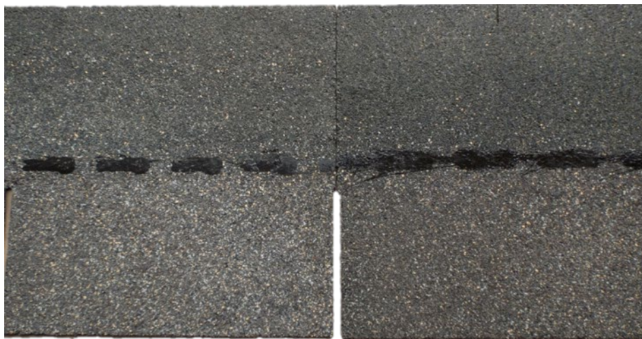
Figure 8-15. Butt Shingles Together on the Upper Part
