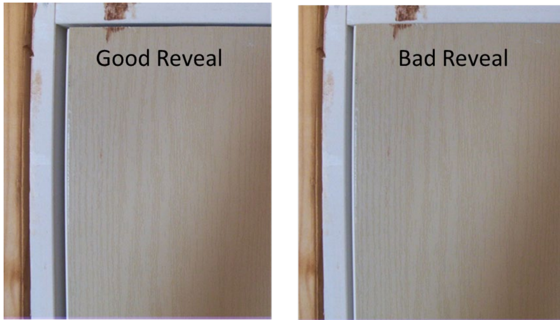
Figure 12-13. Check For Equal Reveals On the Sides and Top of the Door
