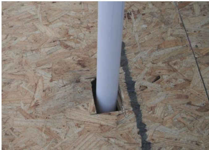
Figure 7-6. Plumbing Vent Stack in Decking
