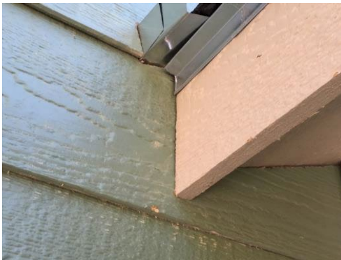
Figure 10-11. Siding at Intersection Wall
