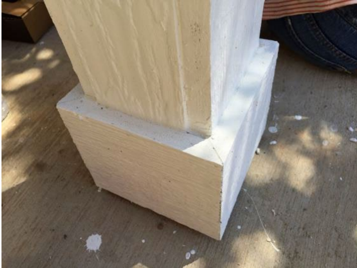
Figure 9-31. Trim at Base of Porch Column
