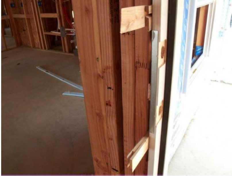
Figure 12-15. Reinforce Door Frame on Strike Side of Jamb
