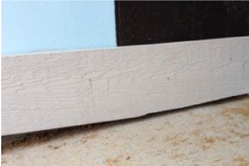
Figure 10-7. Siding on Sloped Porch
