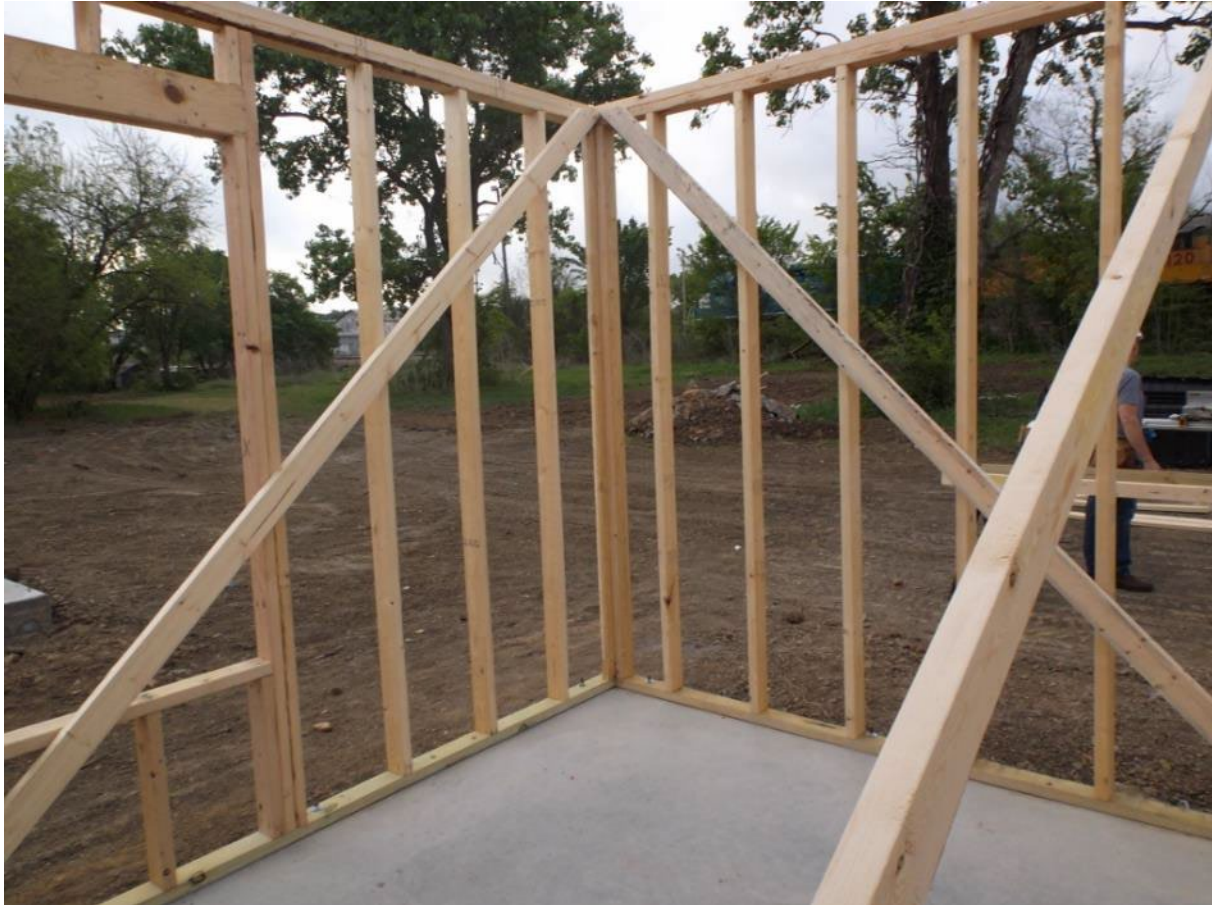
Figure 4-10. Bracing at Exterior Corner
