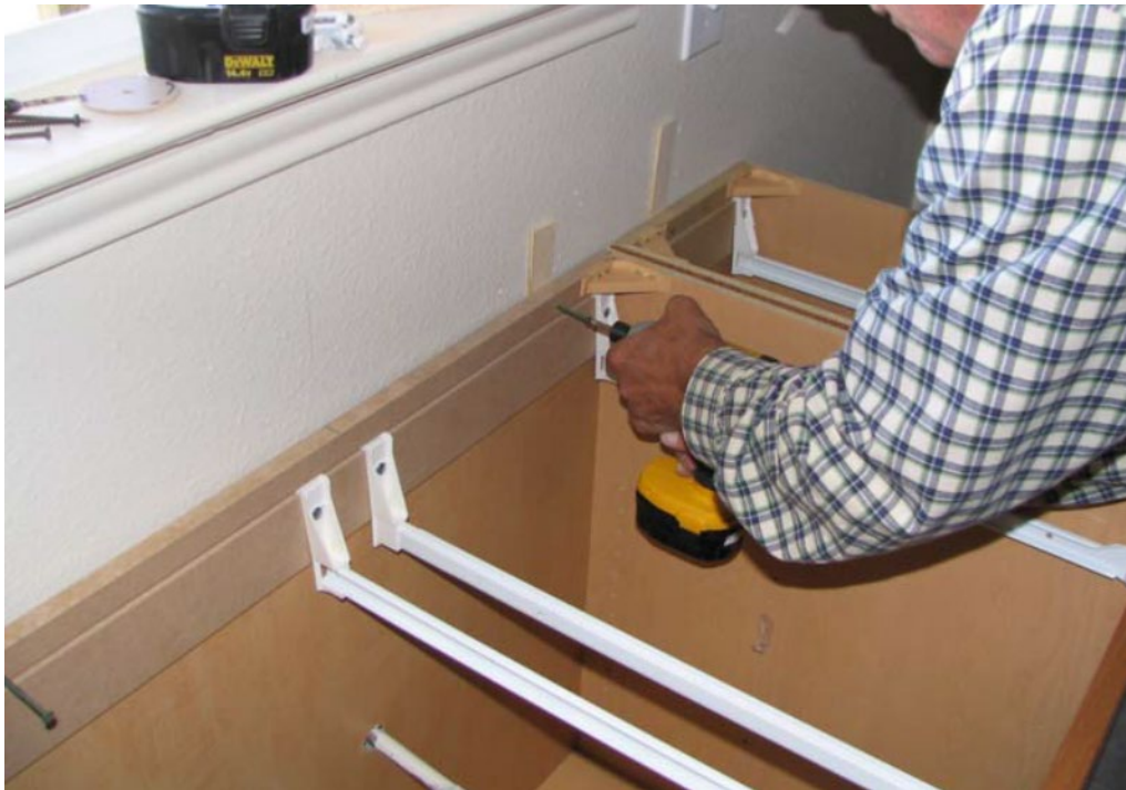
Figure 13-10. Fastening Base Cabinets to the Wall
