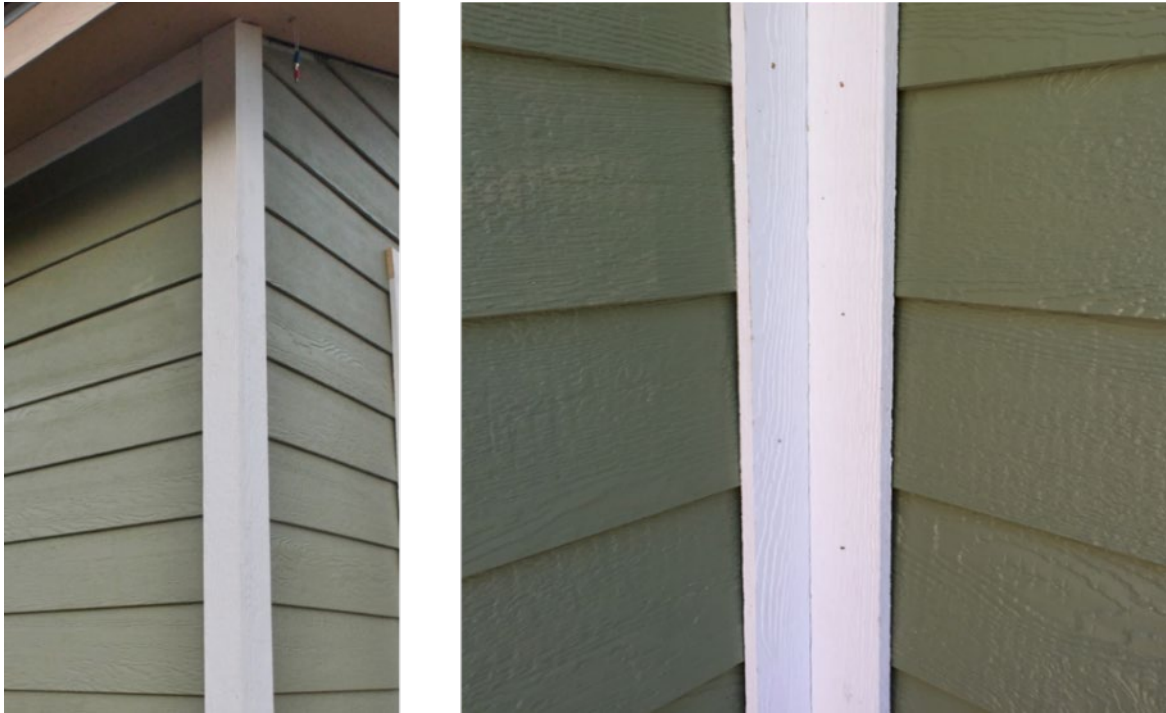
Figure 9-10. Corner Trim - Outside Corner (left) and Inside Corner (right)
