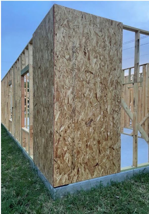
Figure 6-1. Sheathing Detail at Corners
