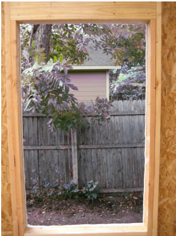
Figure 6-10. Properly Cut Window Opening
