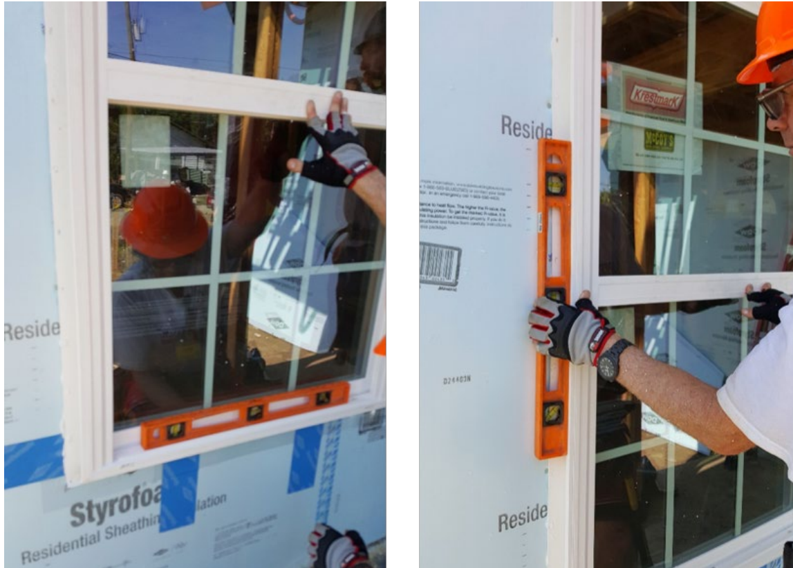
Figure 6-13. Check Fit and Level
