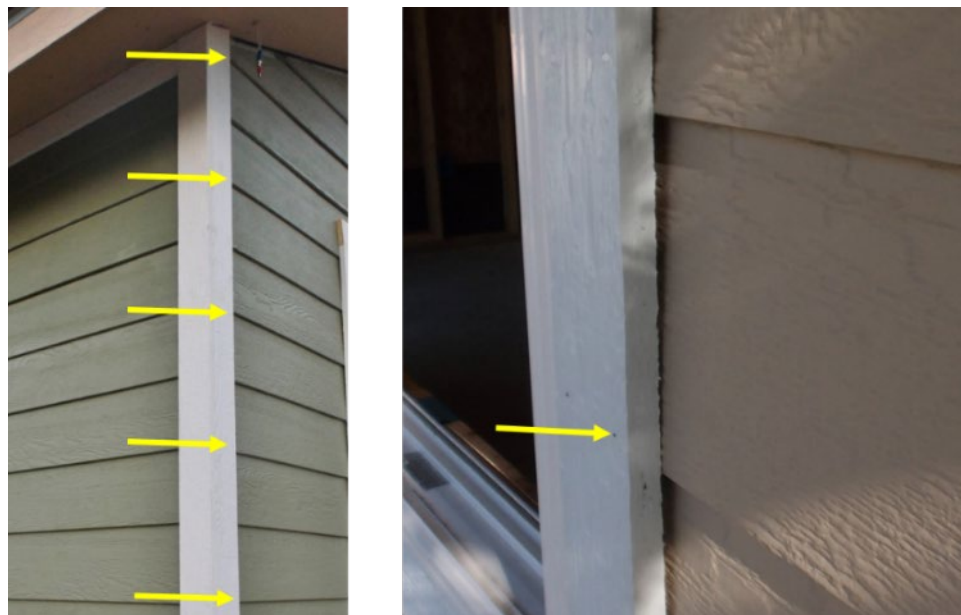
Figure 9-11. Nailing Location for Trim
