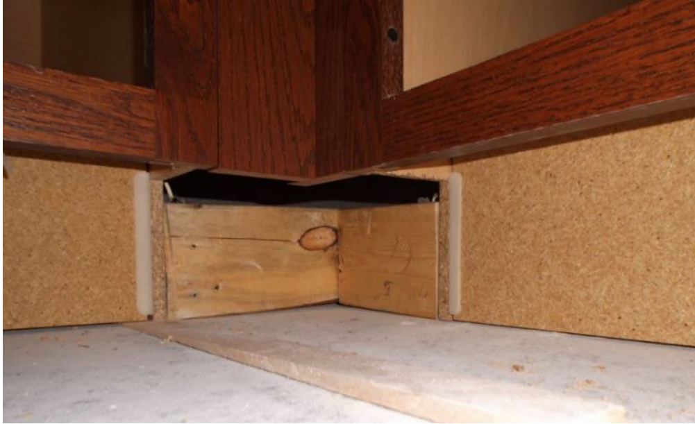
Figure 13-18. Framing for Toe Kick (Front View)
