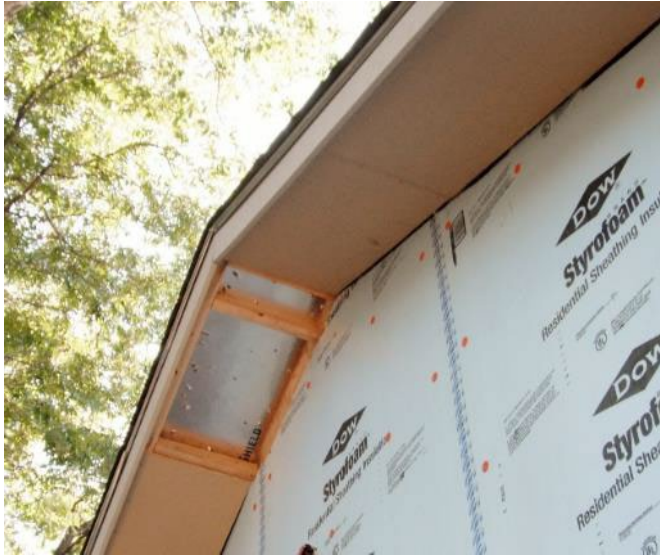
Figure 9-5. Rake Soffit
