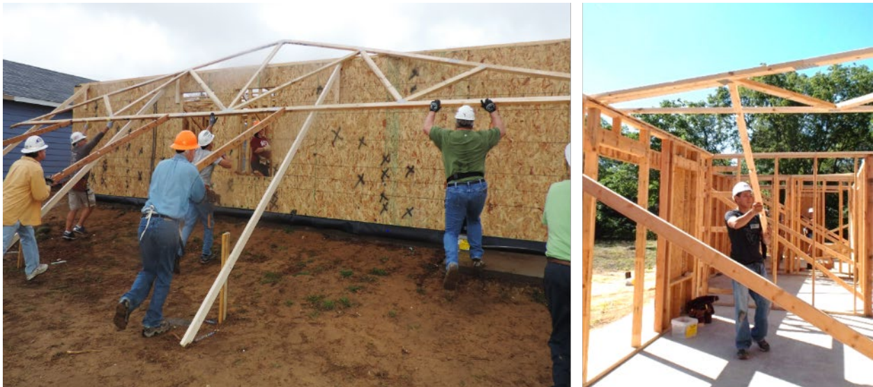
Figure 5-13. Loading Trusses
