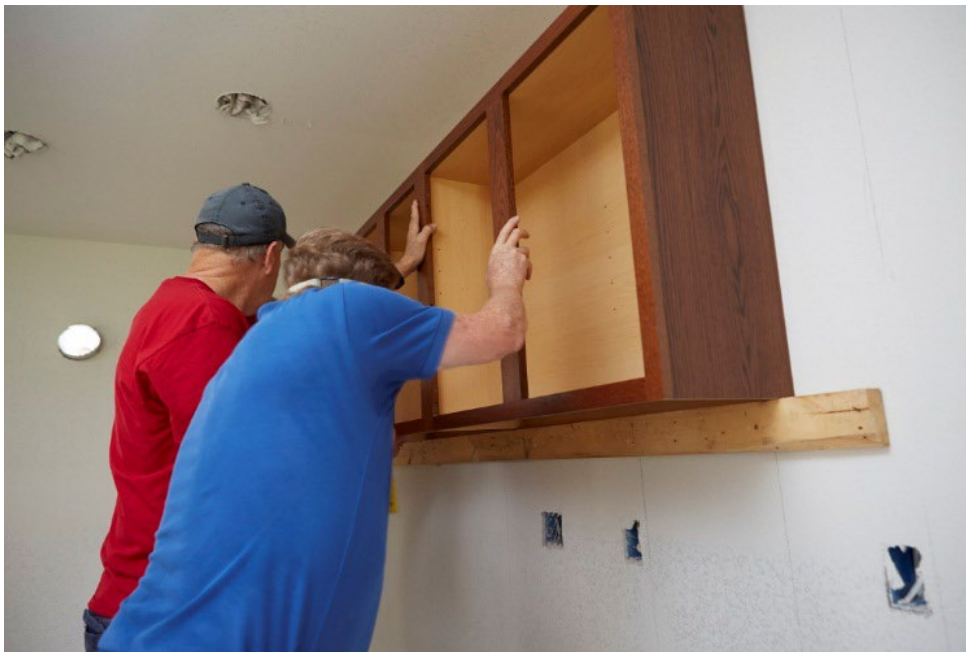
Figure 13-7. Use Cleat to Support Upper Cabinets During Installation
