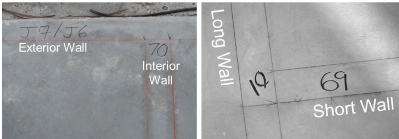
Figure 4-3. Wall Location Markings on Slab
