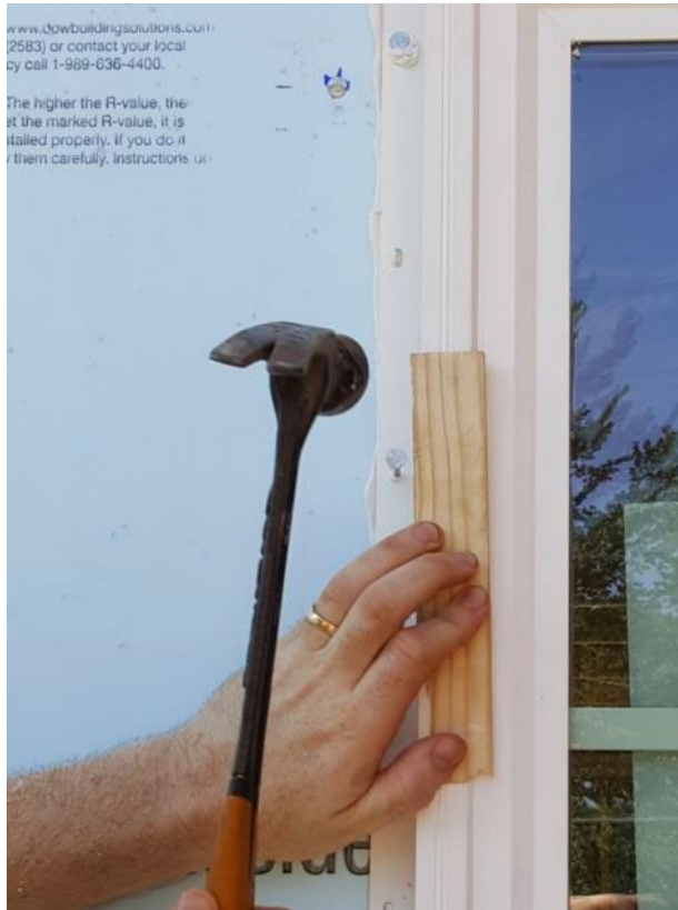
Figure 6-15. Nailing Window in Place
