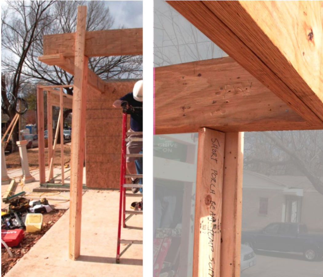
Figure 4-31. Temporary Post for Porch Beam
