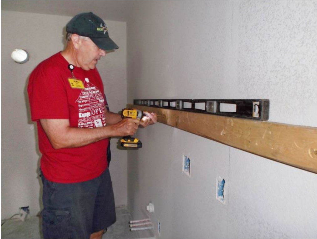
Figure 13-4. Install Cleat to Support Upper Cabinets During Installation
