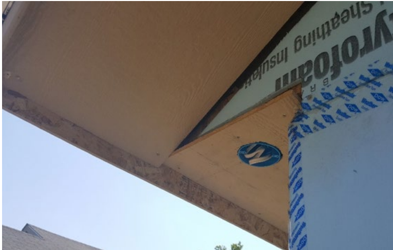
Figure 9-7. Flat Eave Soffit at Rake
