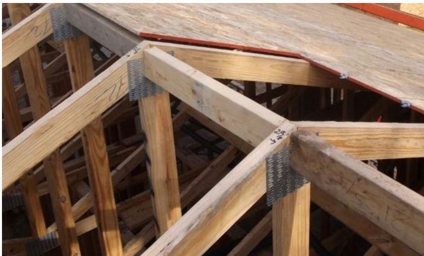
Figure 5-42. Ridge Blocking
