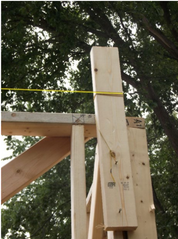
Figure 4-20. Block for Stringing Walls
