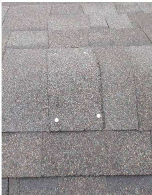
Figure 8-33. Final Piece of Ridge Cap
