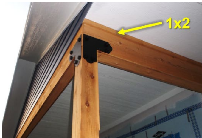
Figure 9-28. Porch Beam Trim at Ceiling and Soffit
