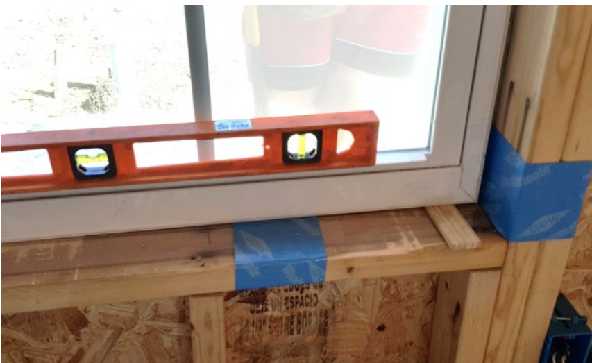
Figure 6-14. Shim Window as Needed
