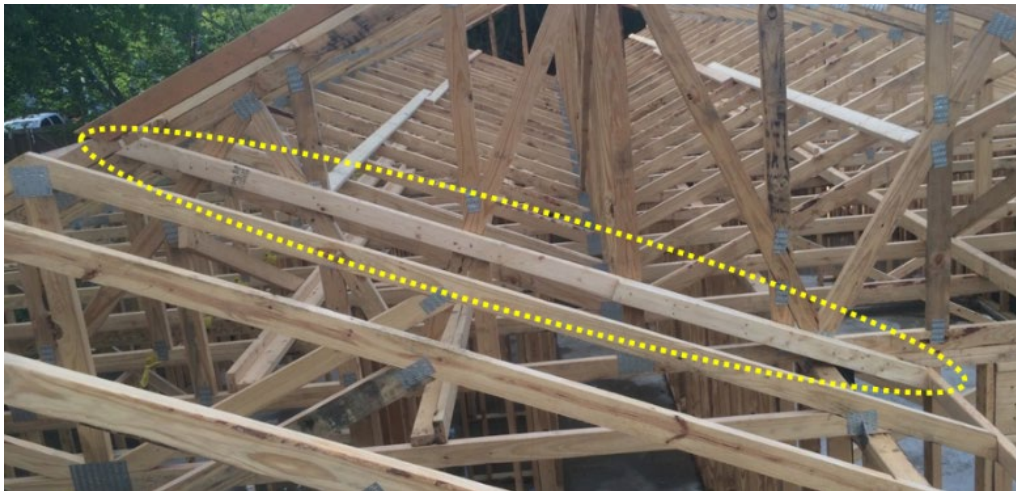
Figure 5-15. Mark for Decking Nailer Before Setting Smaller Trusses
