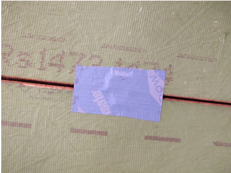
Figure 7-7. Apply 2-Inch Square of Butyl Tape over Each H-Clip
