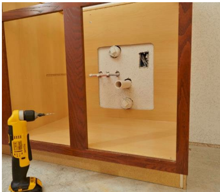
Figure 13-12. Plumbing Cutouts Using a Jigsaw
