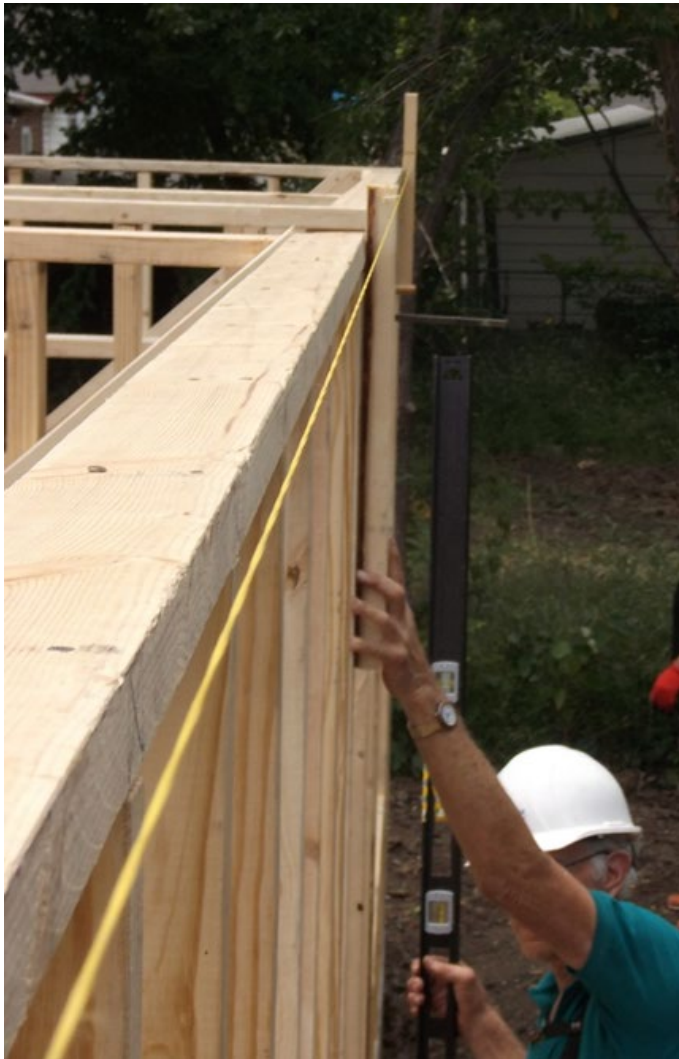
Figure 4-21. Using 2x4 to Help Plumb Exterior Walls
