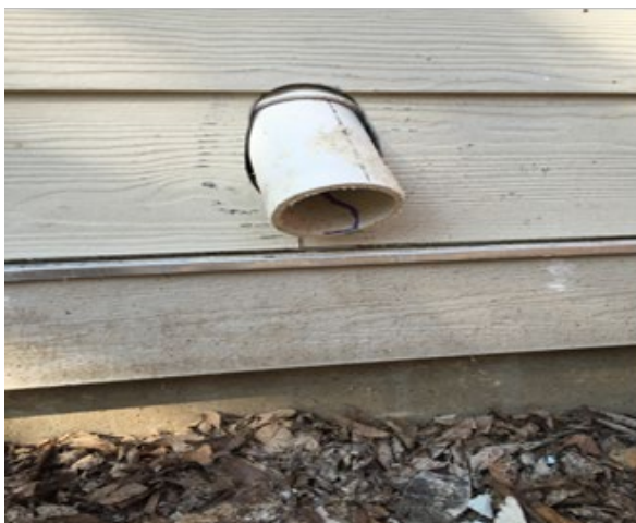
Figure 10-4. Siding Cut Outs for Protrusions
