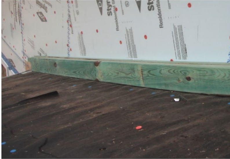
Figure 8-23. Brick Ledger Board
