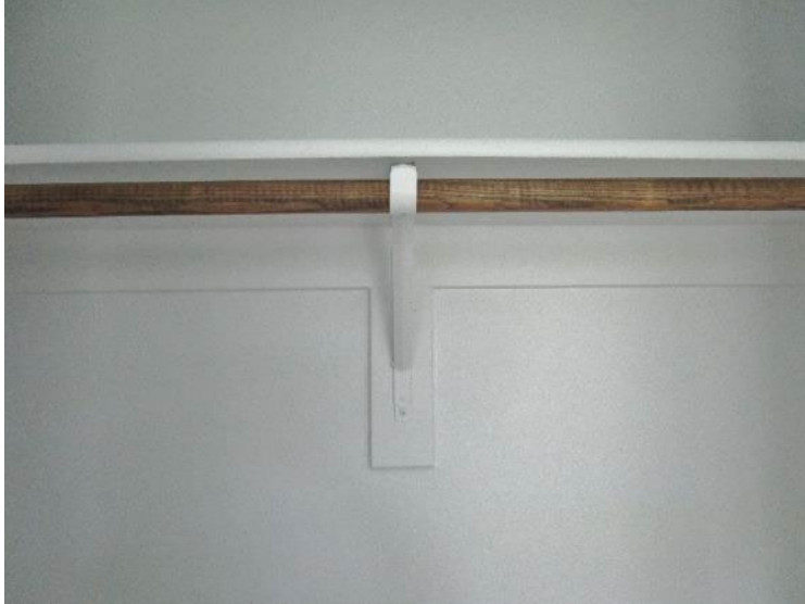
Figure 12-23. Shelf Bracket Support
