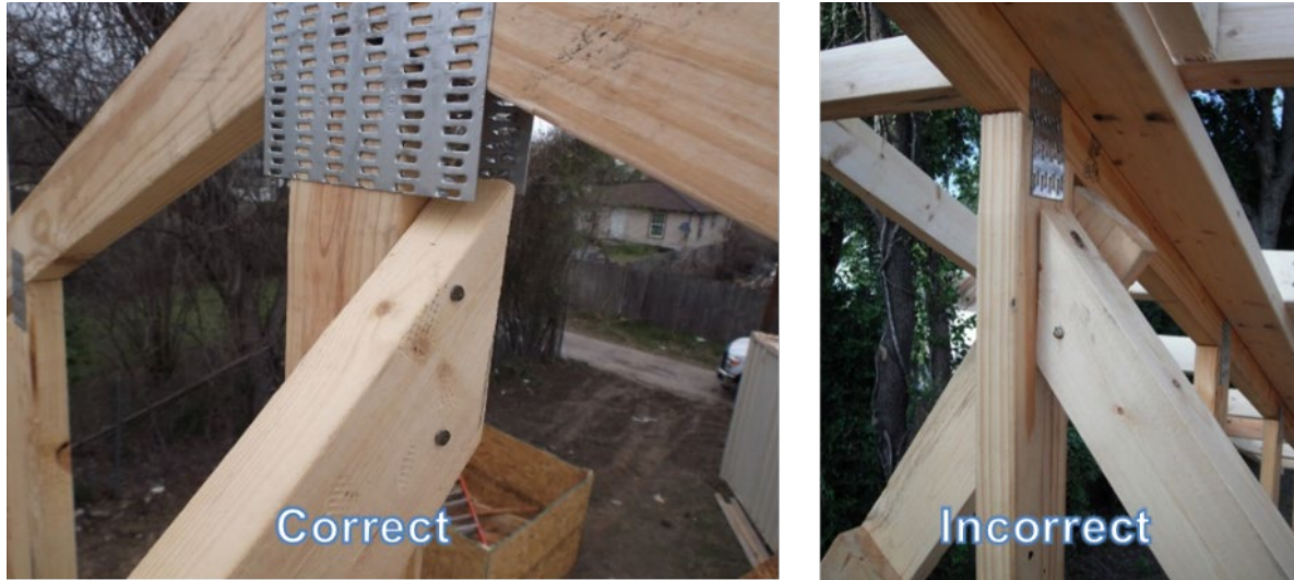
Figure 5-22. K-Bracing Connection at Truss
