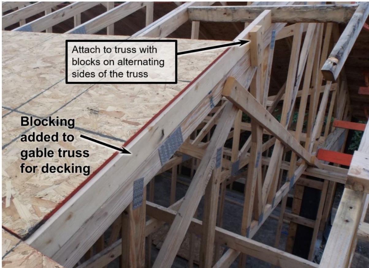
Figure 5-41. Blocking Added to Gable Truss for Decking
