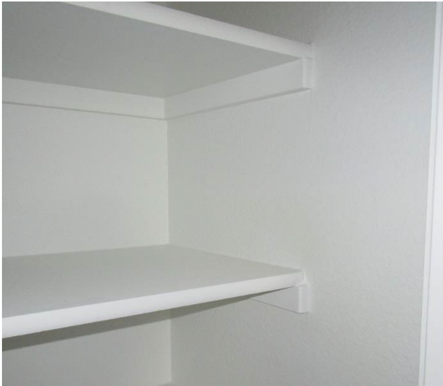
Figure 12-22. Support Brackets for Shelving
