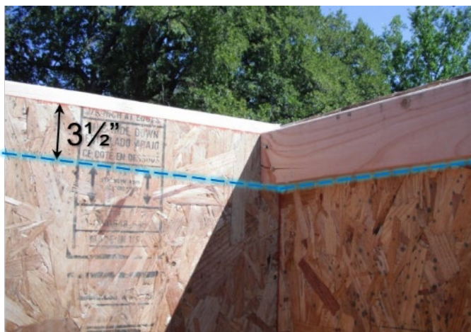
Figure 4-46. Ledger Boards for HVAC Closet Ceiling
