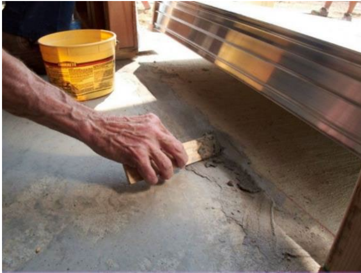
Figure 12-3. Filling Large Gap Under the Threshold
