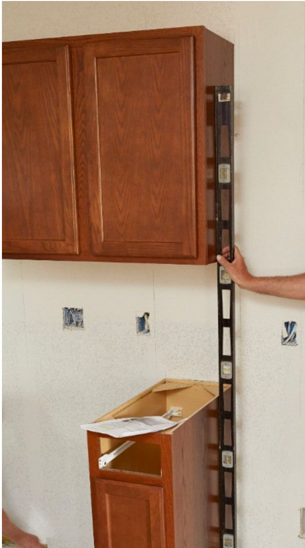
Figure 13-9. Base Cabinet Should be Plumb (Even) with the Upper Cabinet
