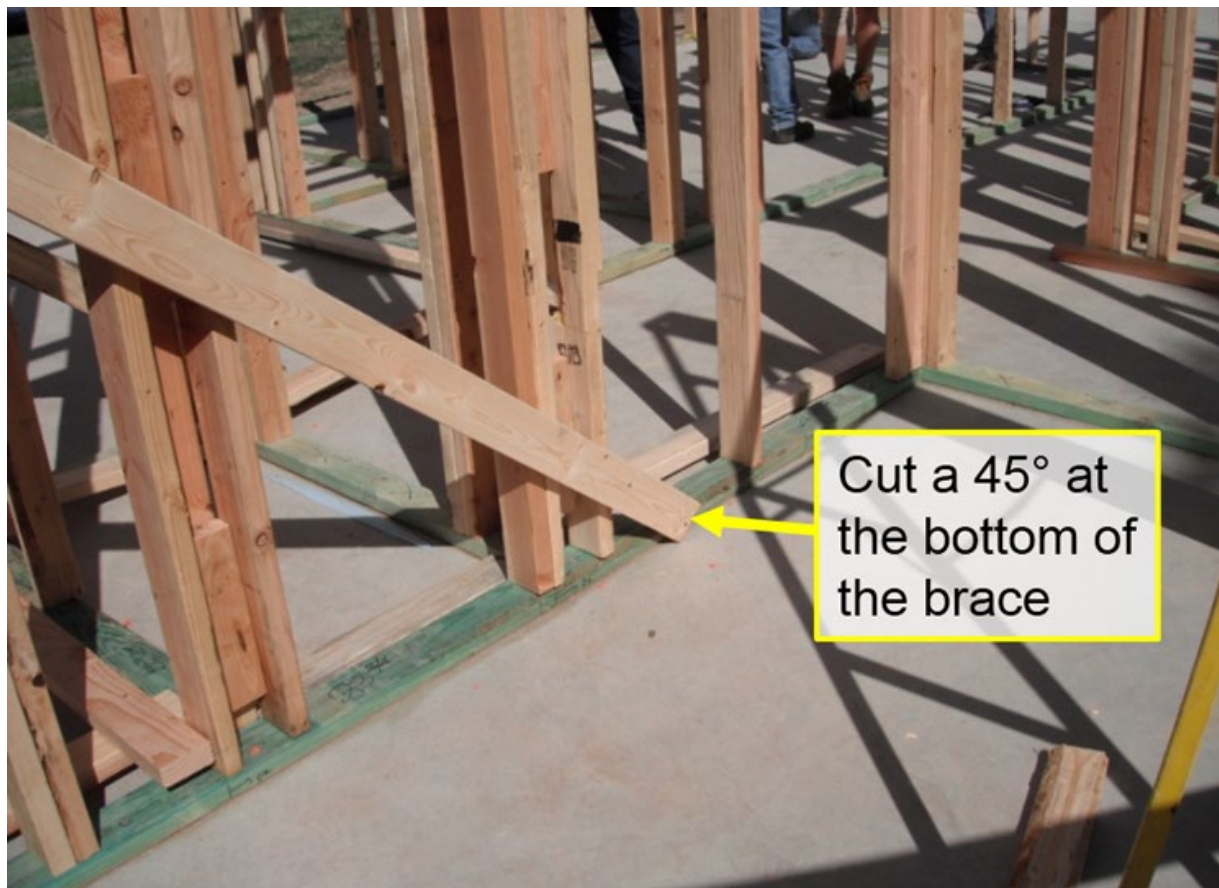
Figure 4-9. Wall Bracing
