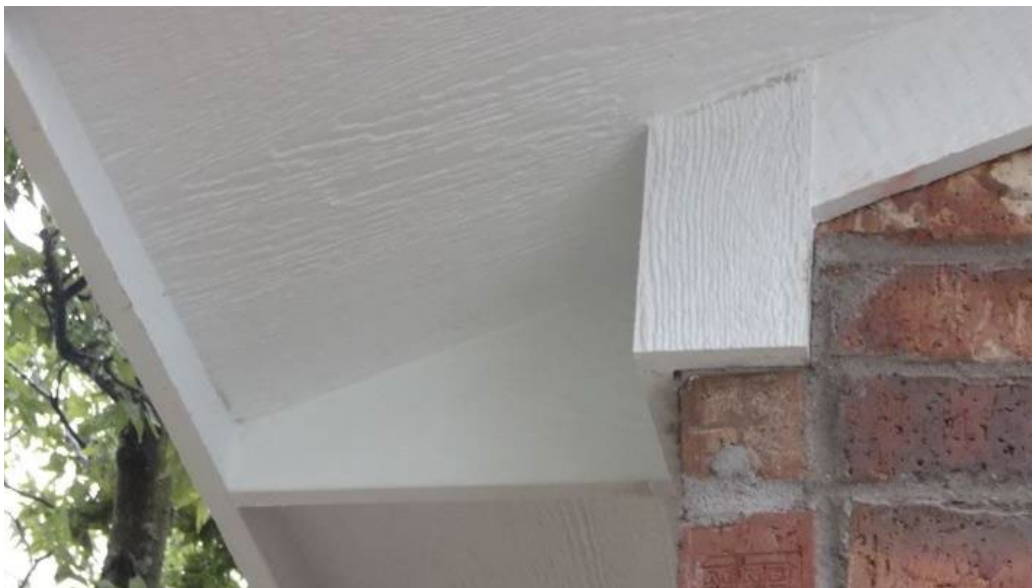
Figure 9-23. Installed Bird Box (Brick-to-Brick Transition), Option 1
