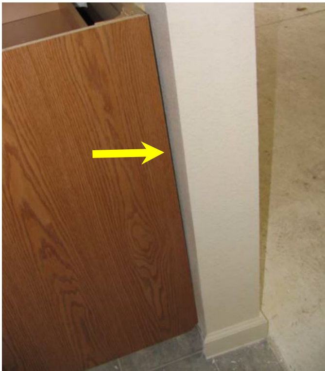
Figure 13-21. Add Scribe Molding to Cover Gap
