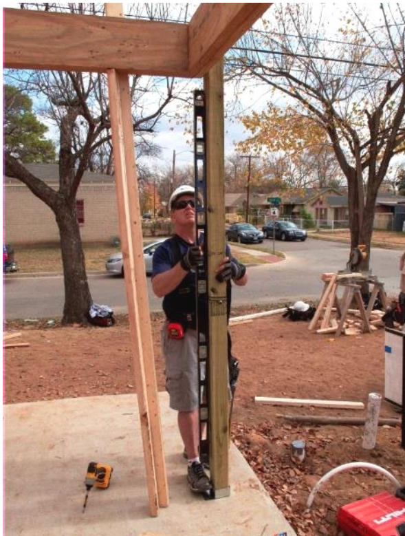
Figure 4-34. Locating Porch Post on Slab
