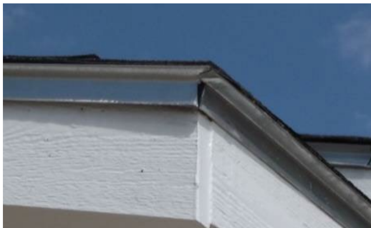
Figure 8-5. Installed Drip Edge at Corner
