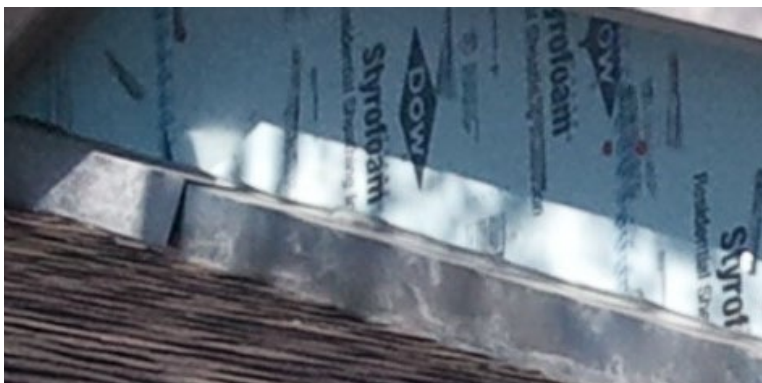
Figure 8-25. Brick Ledger Board Flashing
