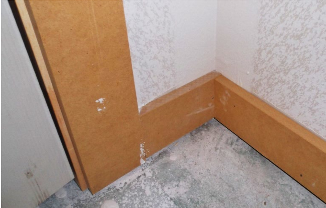
Figure 12-16. Baseboard Inside Corner Joint
