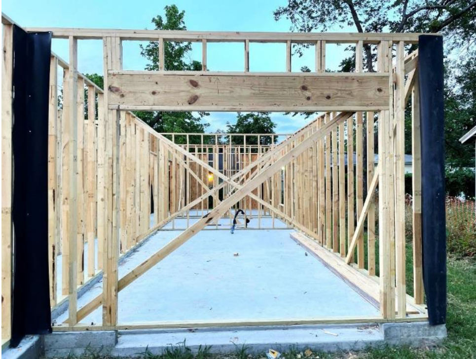
Figure 4-18. Completed and Installed Garage Door Wall with Bracing
