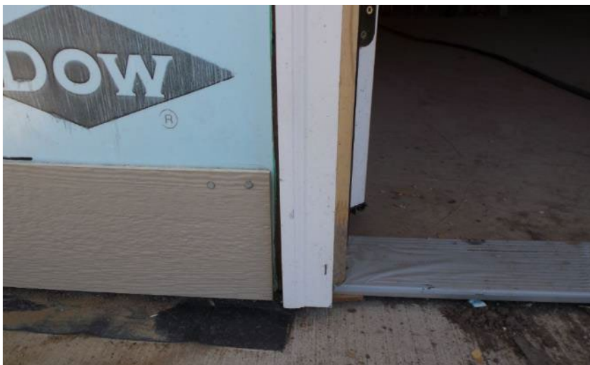
Figure 10-10. Siding Around Doors
