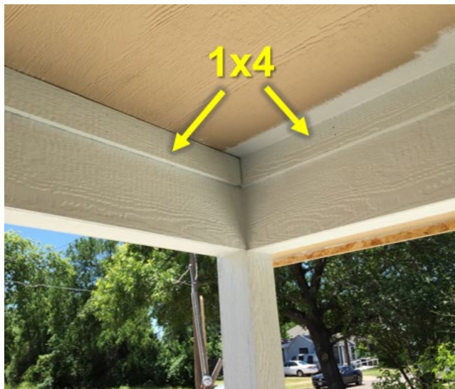
Figure 9-27. Porch Beam Trim at Ceiling and Soffit
