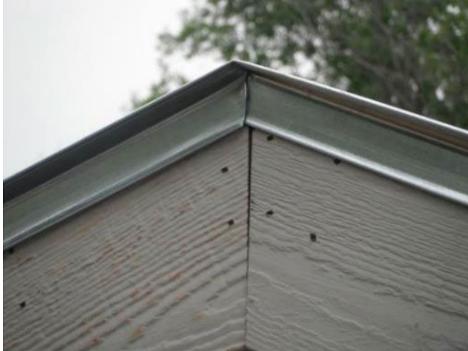
Figure 8-7. Drip Edge over Peak
