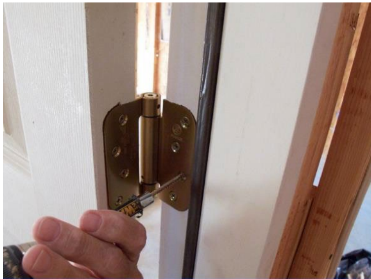
Figure 12-14. Replace One of the Hinge Screws with a Long Screw
