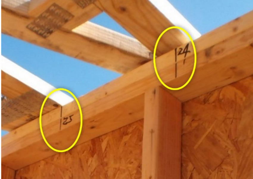
Figure 5-7. Truss Location Labeled on Cap/Top Plates
