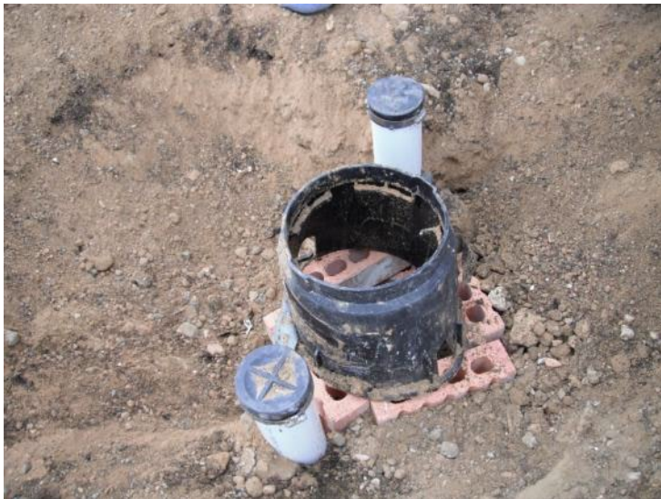
Figure 15-3. Resetting Level of Valve Box
