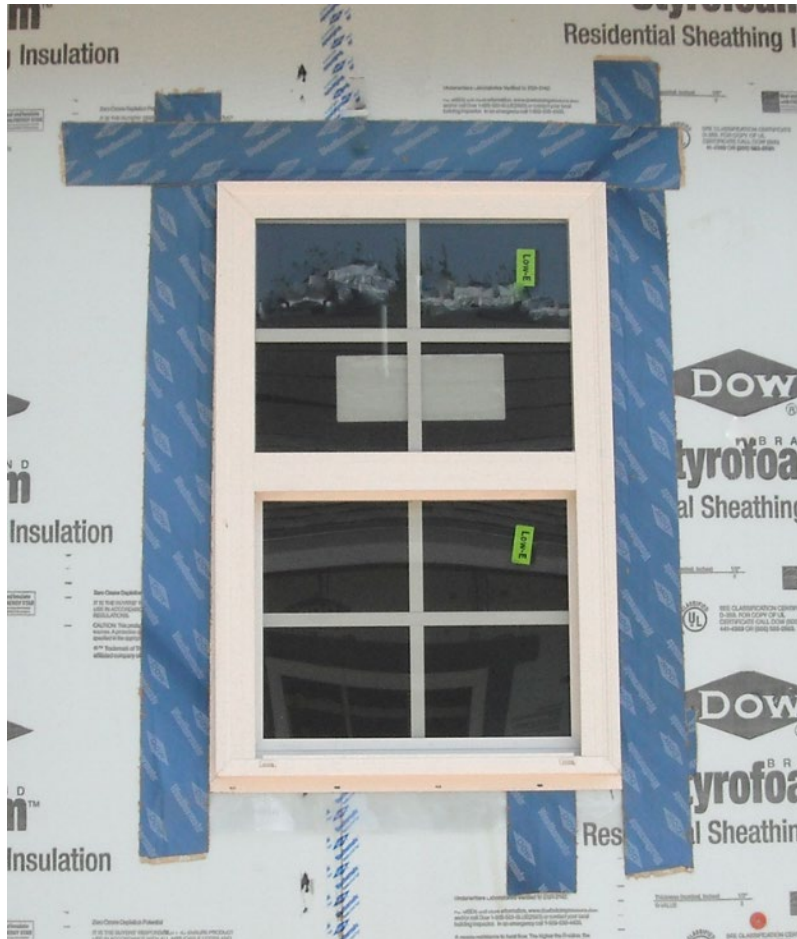
Figure 6-16. Install Butyl Adhesive Tape Around Sides and Top of Window
