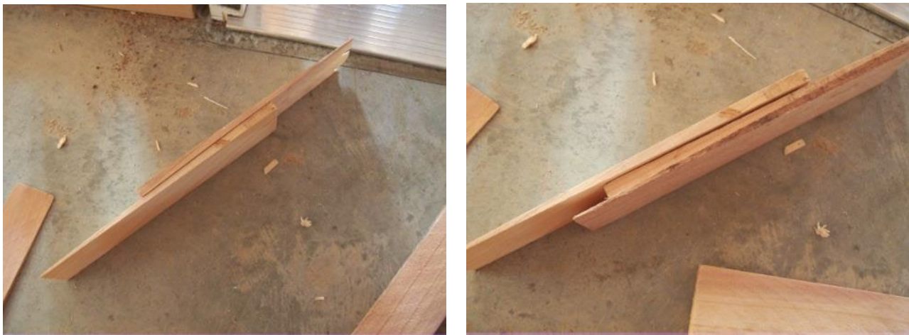
Figure 12-10. Use Shims in Pairs
