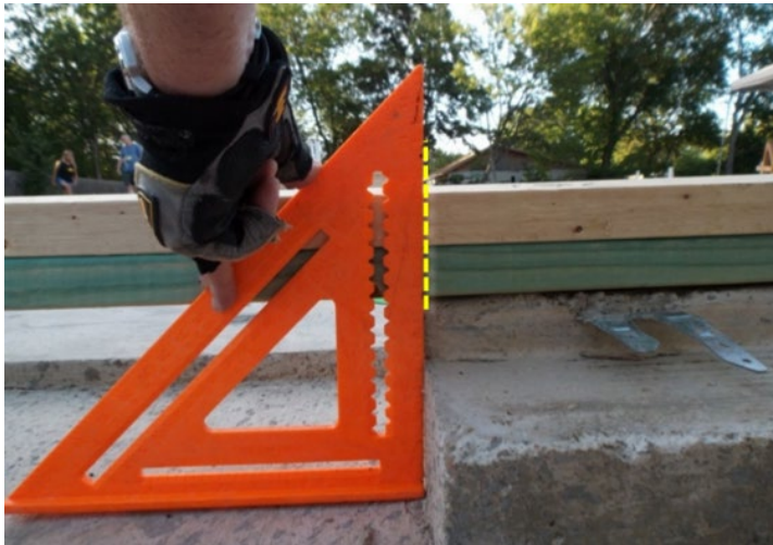
Figure 4-15. Marking the Plates for the Garage Door Opening
