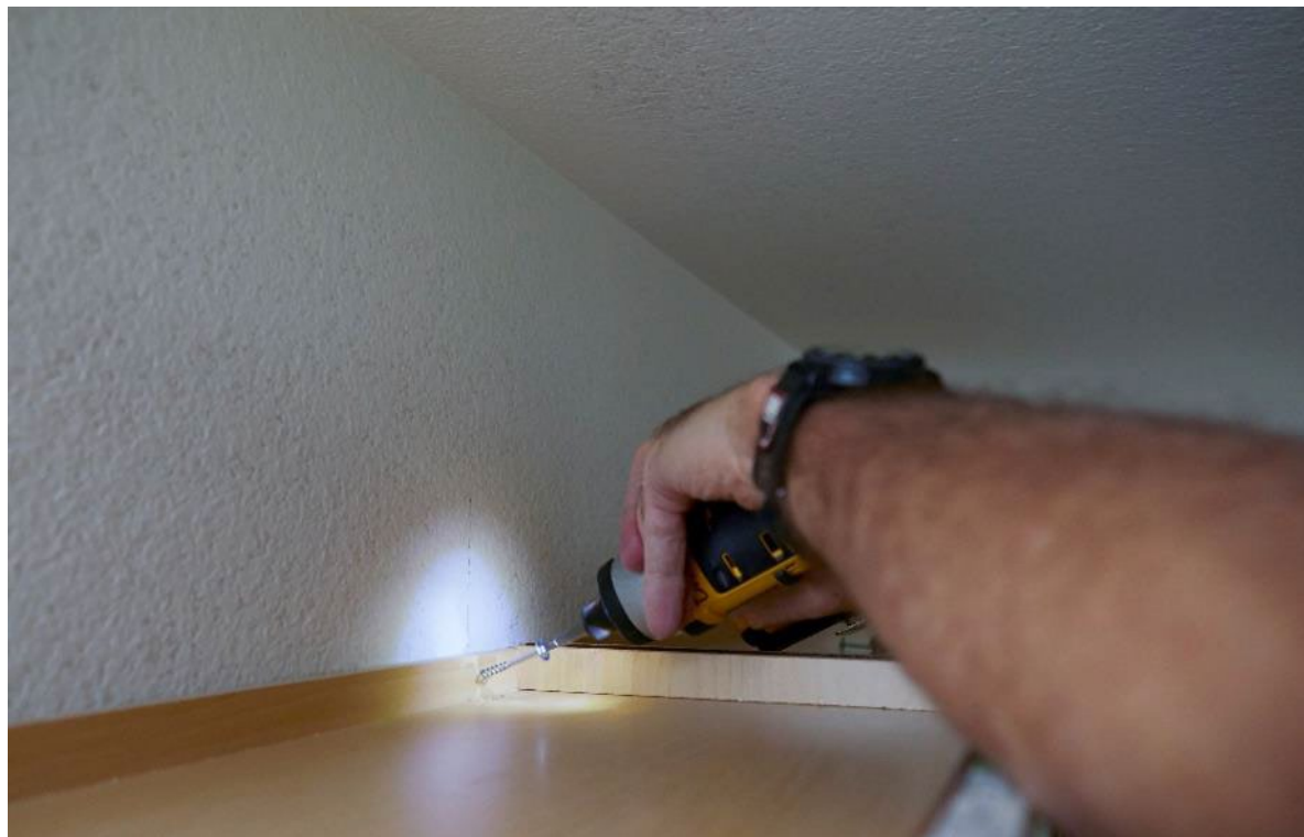
Figure 13-8. Securing Top of Upper Cabinets to Wall
