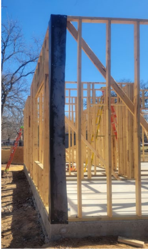
Figure 4-39. Installation of Poly at Corners
