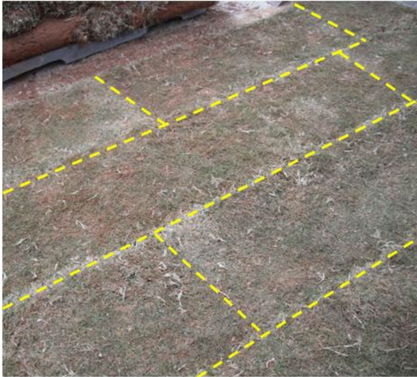
Figure 15-2. Lay Sod With Staggered Seams
