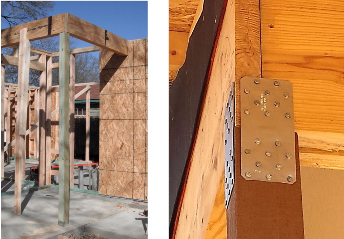
Figure 4-38. Installed Porch Post with Simpson Nail Plate
