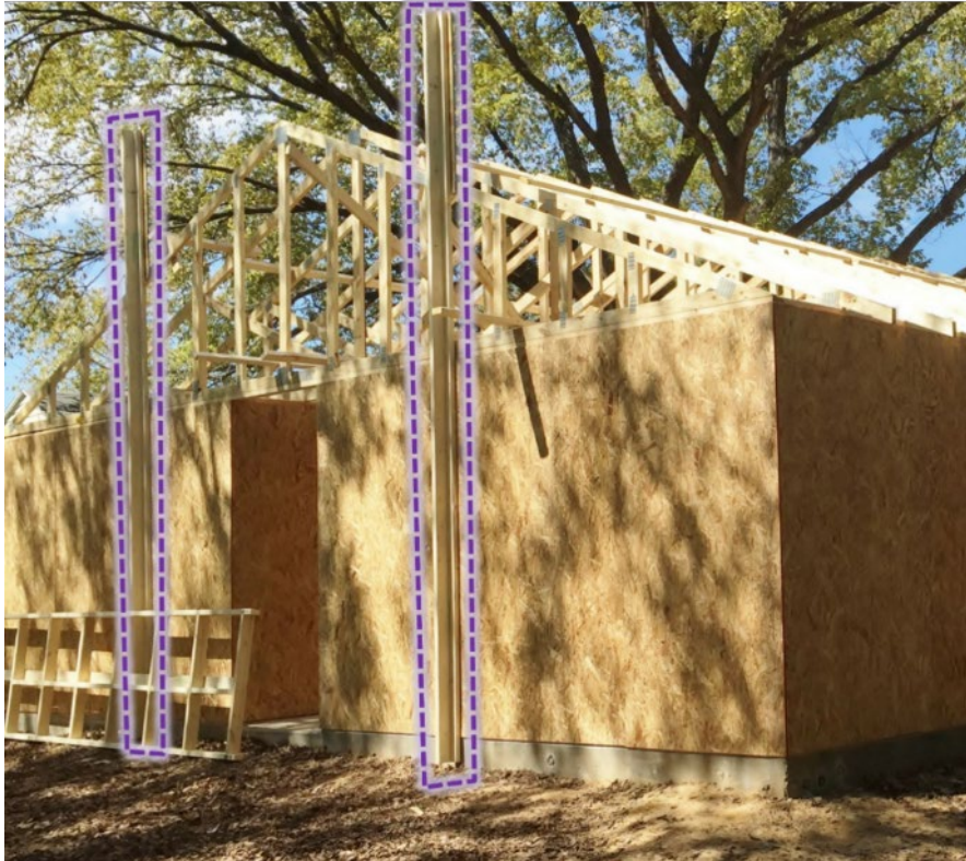
Figure 5-17. Strongback (Highlighted in Purple) Bracing of Back Gable Truss
