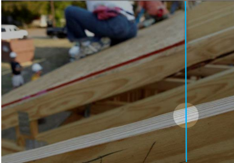
Figure 7-3. Chalk Line for First Row of Decking
