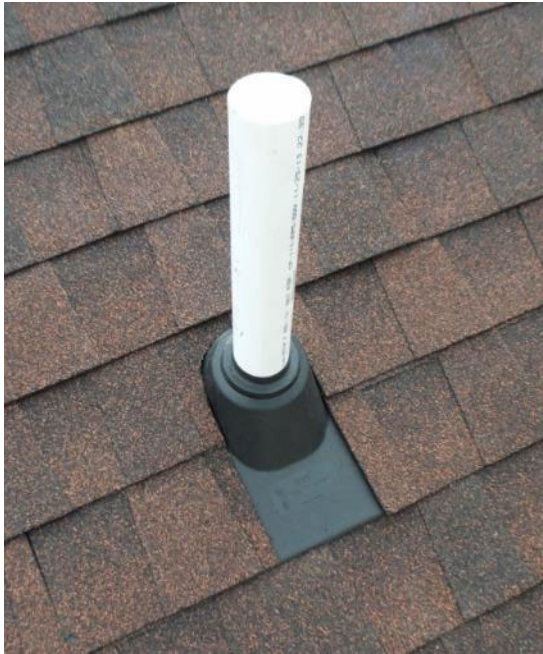
Figure 8-28. Cut Shingle(s) to Fit Around the Boot
