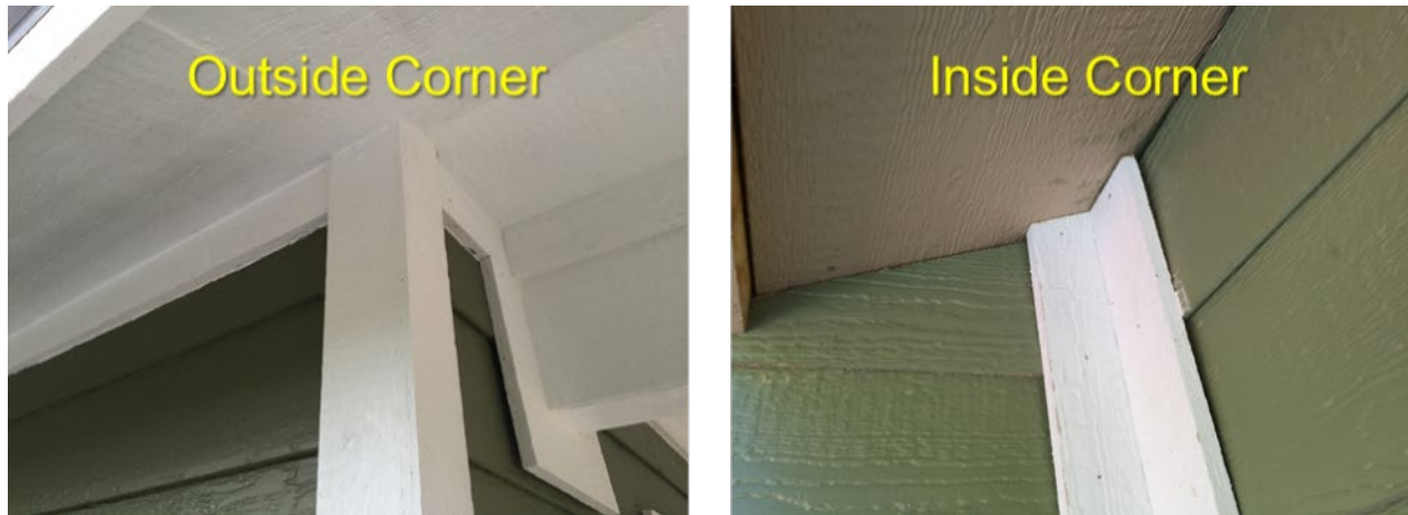
Figure 9-12. Corner Trim at Soffit
