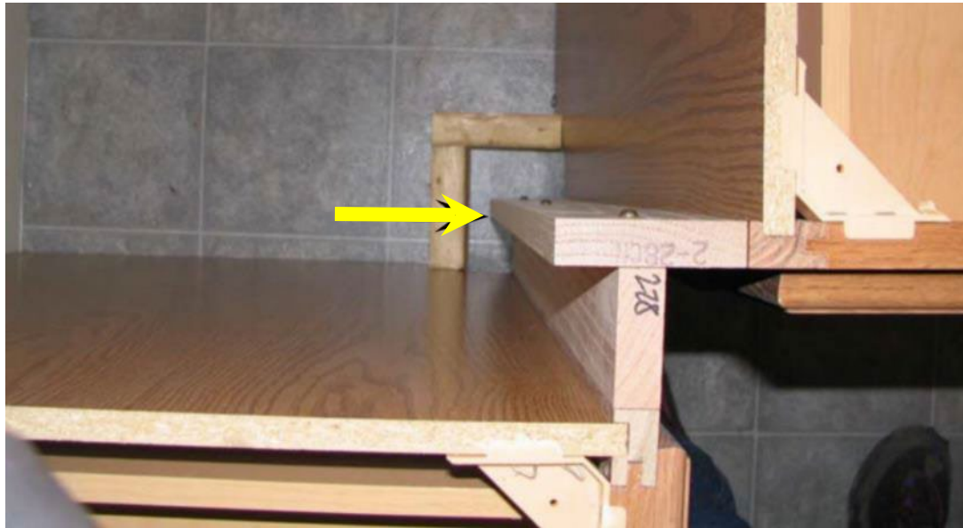
Figure 13-15. Connecting Filler Strips (Top View)
