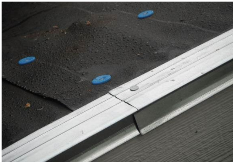
Figure 8-6. Placement of Drip Edge on the Rake
