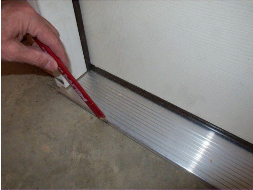
Figure 12-7. Mark Location of Threshold on Slab
