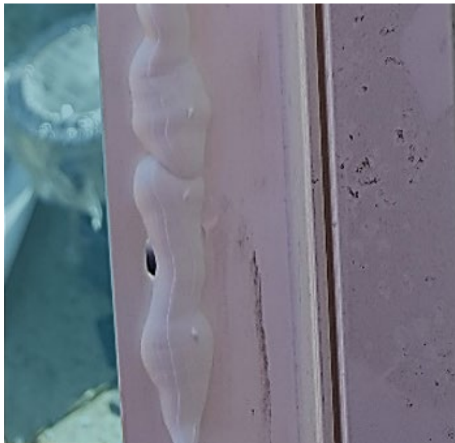
Figure 6-12. Caulk the Inside Flange of the Window
