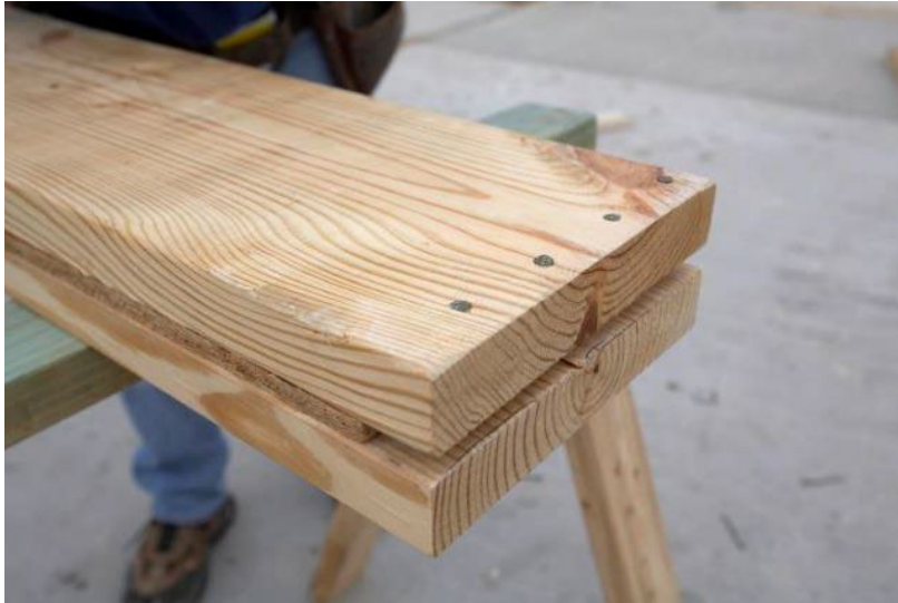
Figure 4-16. Garage Door Header Using 2x12 Lumber
