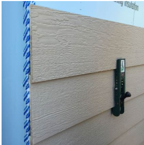
Figure 10-6. Using Siding Gauges to Maintain 7-Inch Reveal
