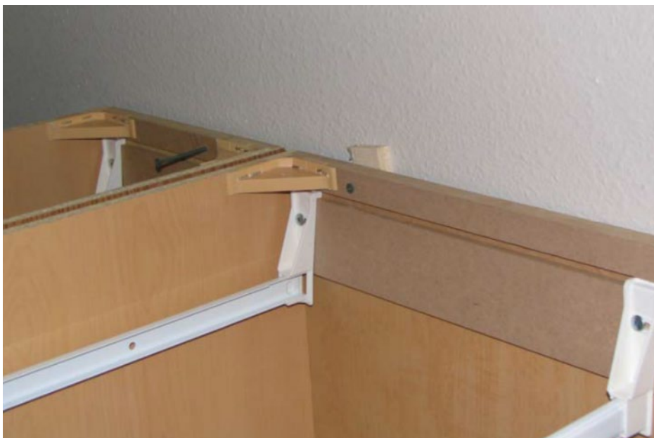
Figure 13-14. Use Shims to Prevent Bowing the Cabinets
