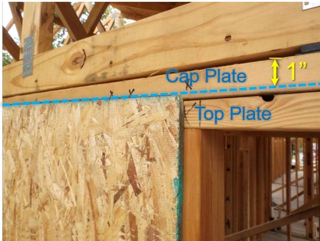
Figure 6-2. Wall Sheathing Set 1-Inch Below the Top of the Cap Plate
