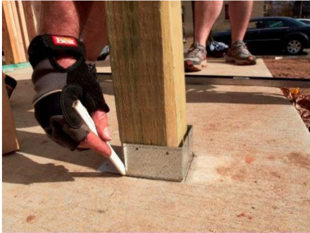
Figure 4-35. Marking Location of Porch Post on Slab
