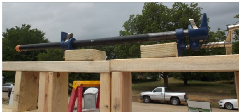
Figure 4-8. Nailing Pattern for Connecting Walls, Clamping as Needed
