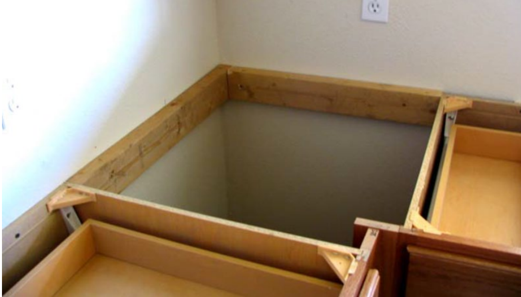
Figure 13-16. Framing for Counter Top in Corners
