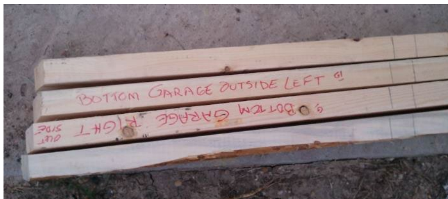
Figure 5-29. Mark the Ultimate Location on the Ladder Panels
