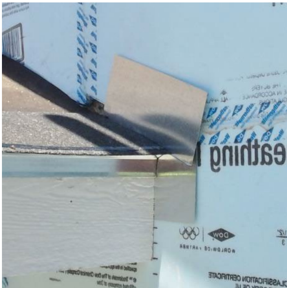
Figure 8-2. Kick-Out Flashing Placement at Siding Wall
