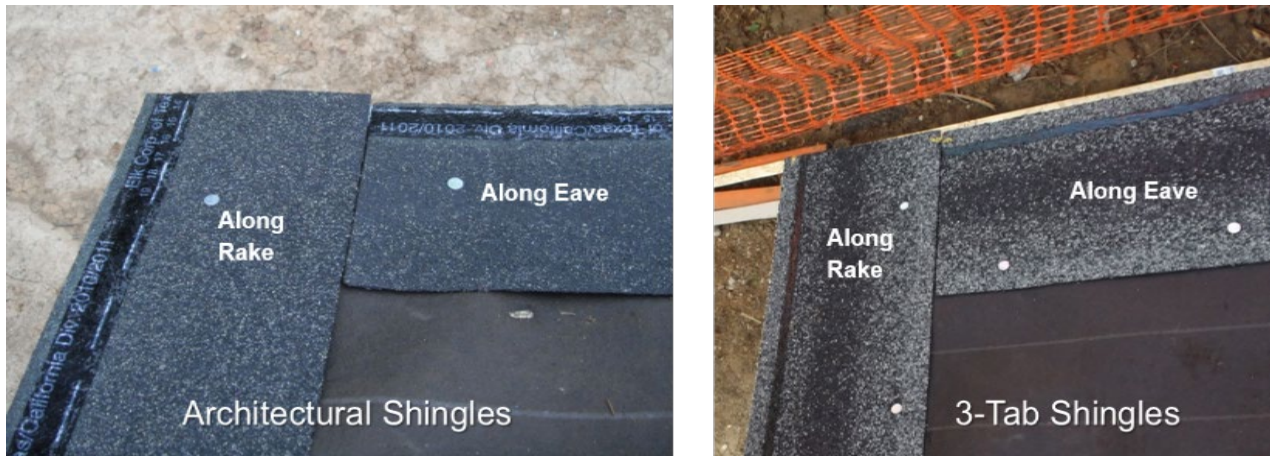
Figure 8-9. Starter Strip at Corner
