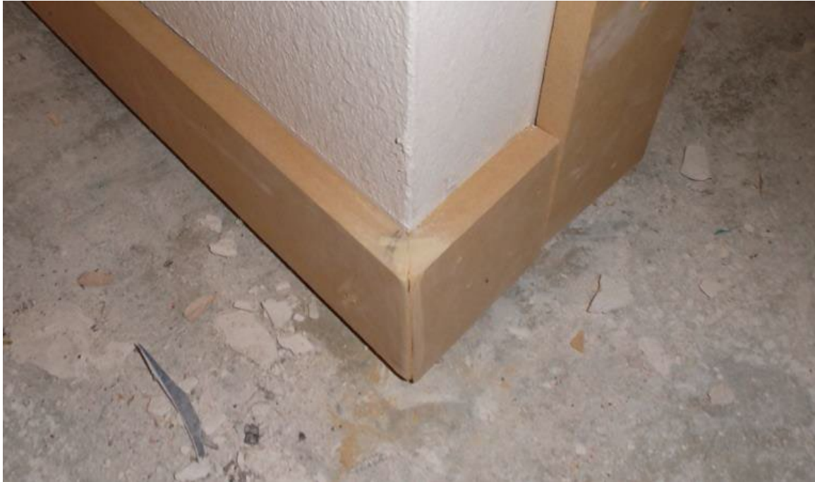
Figure 12-18. Installed Baseboard (Outside Corner)
