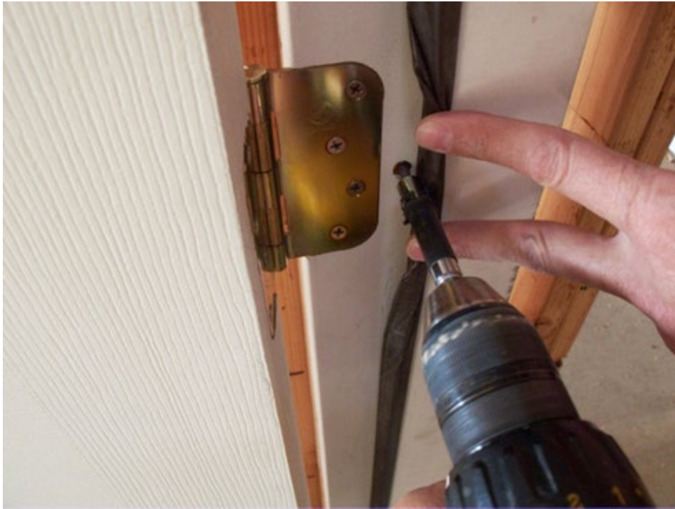
Figure 12-9. Fold Back Weather Stripping to Install Screws
