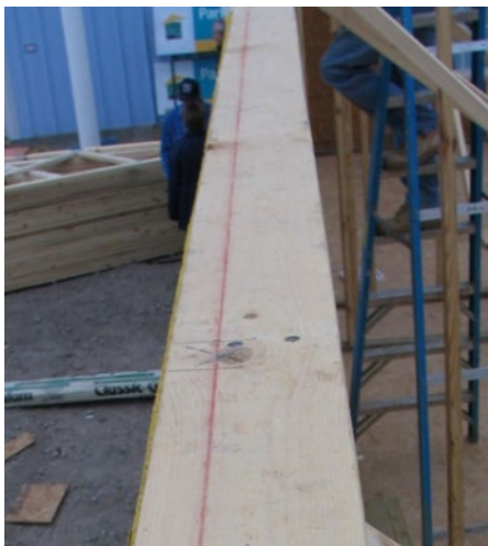
Figure 5-8. Chalk Line on Top of Cap Plate
