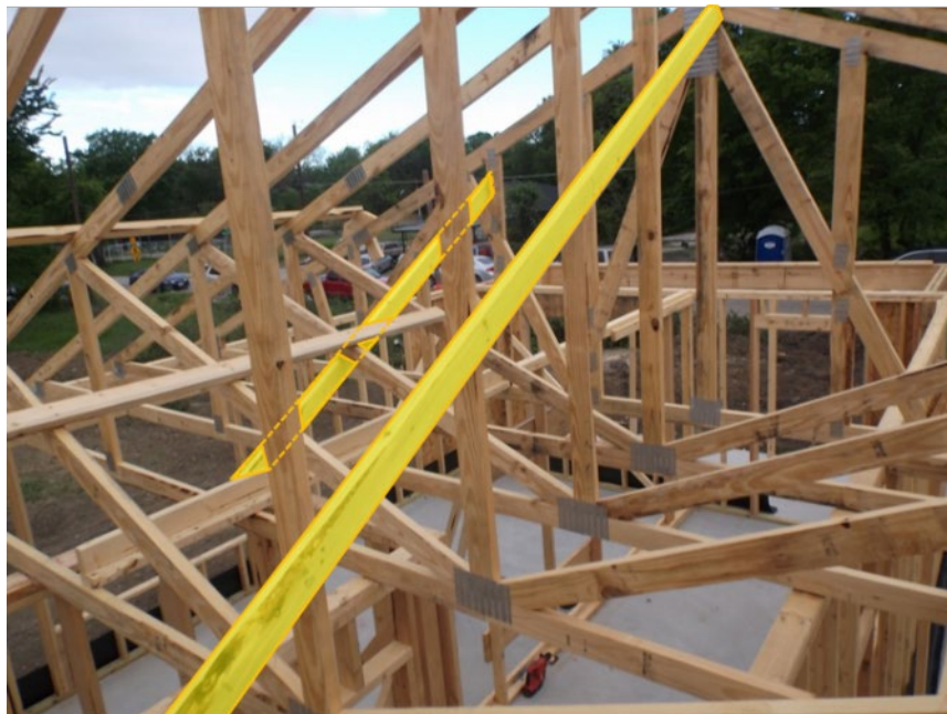
Figure 5-23. K-Bracing Attached to King Post (right), California Corner (left)
