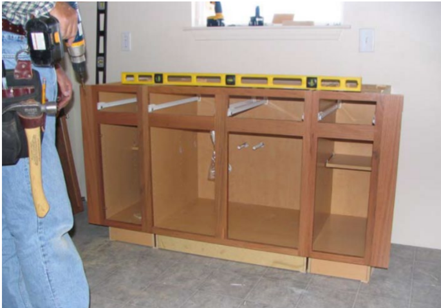
Figure 13-13. Check Level of Base Cabinets
