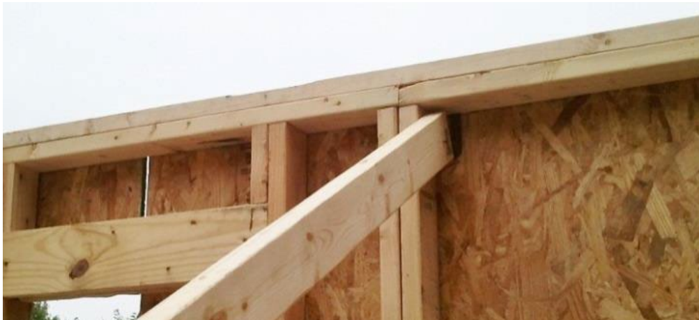
Figure 4-23. Cap Plate on Long Wall
