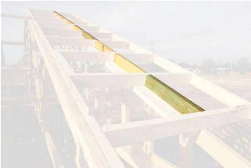
Figure 5-37. Ladder Panel Blocking Placement
