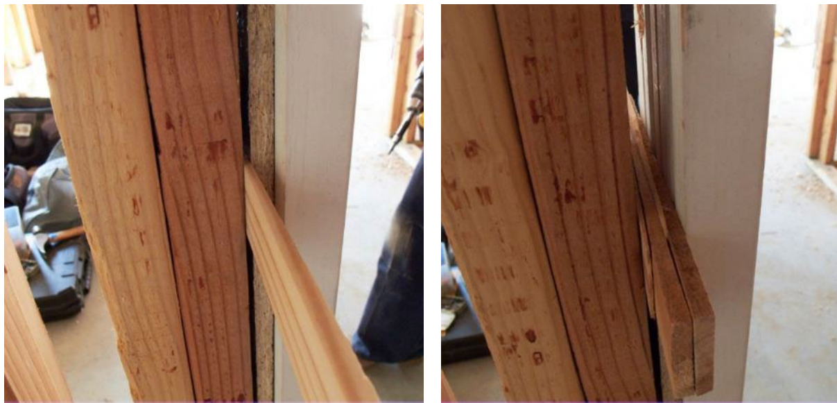
Figure 12-12. Use Shims to Adjust the Reveal
