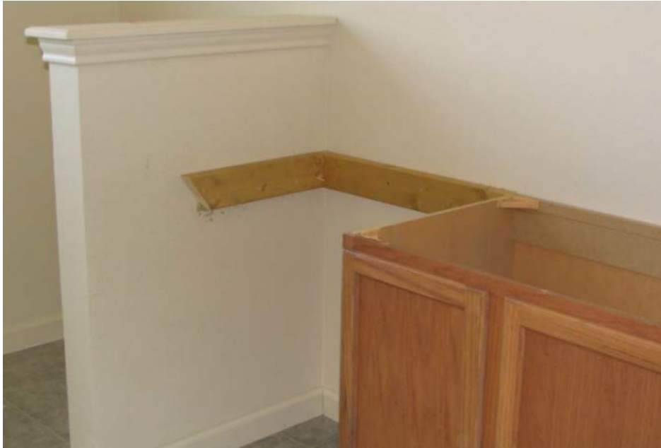
Figure 13-19. Bathroom Countertop Support
