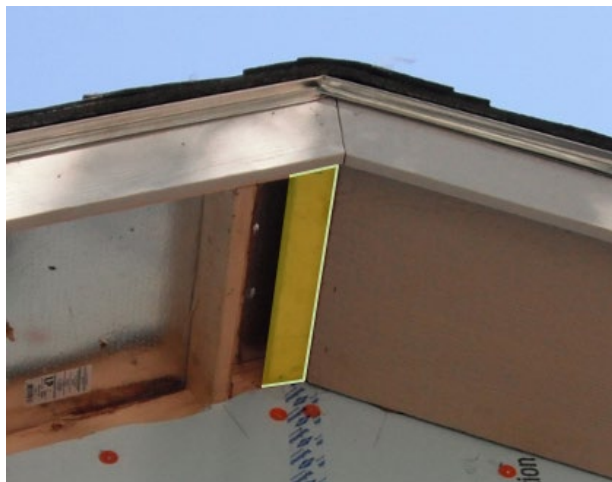
Figure 9-6. 2x4 (Highlighted in Yellow) Installed at Peak to Provide Nailing Surface
