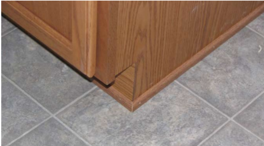
Figure 13-20. Kick Plates and Shoe Molding Around Base Cabinet
