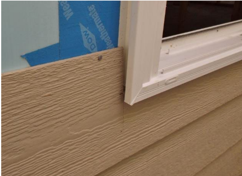
Figure 10-9. Siding Around Windows
