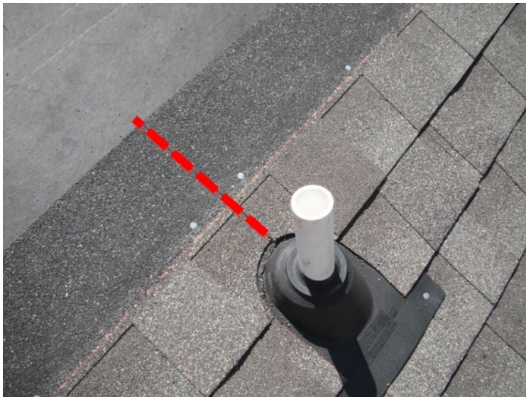
Figure 8-29. Avoid a Seam Directly Over the Boot
