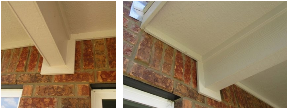
Figure 9-19. Brick Frieze around Porch Beam Covered with Trim
