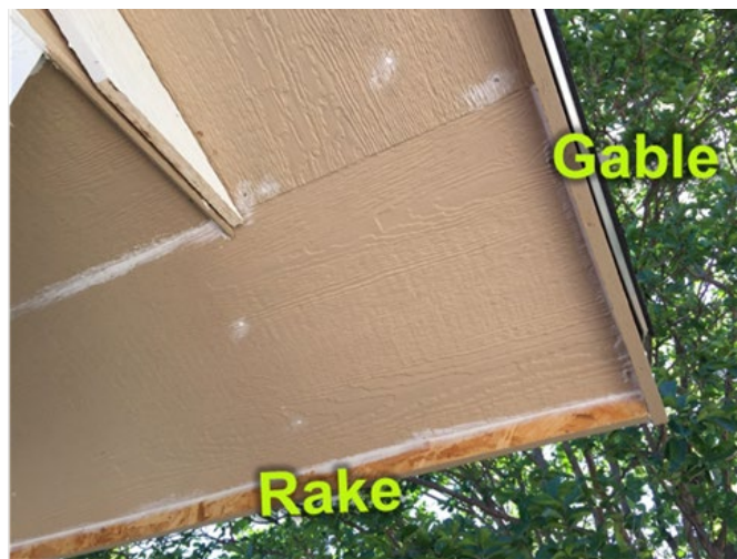
Figure 9-8. Sloped Eave Soffit at Rake
