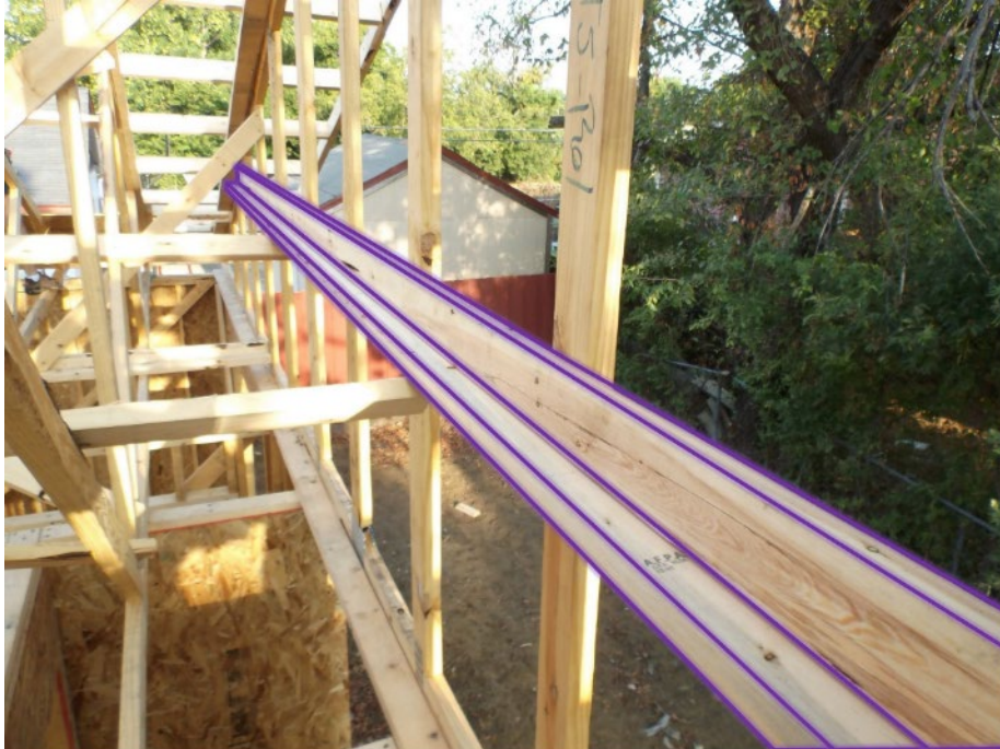
Figure 5-27. Back Gable Horizontal Bracing
