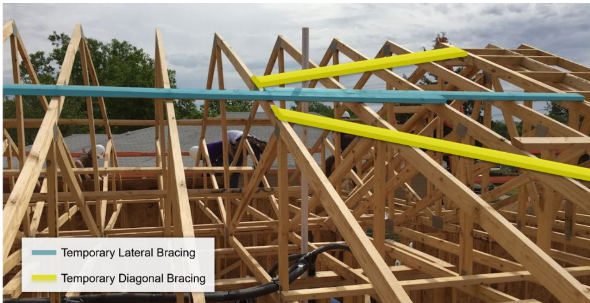
Figure 5-20. Temporary Truss Bracing
