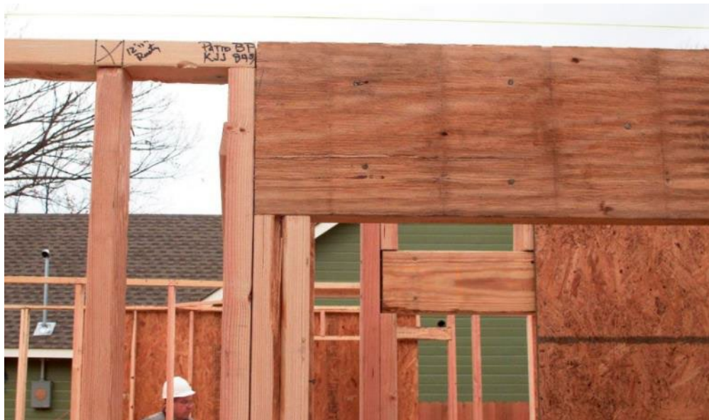
Figure 4-27. Installed Side Porch Beam
