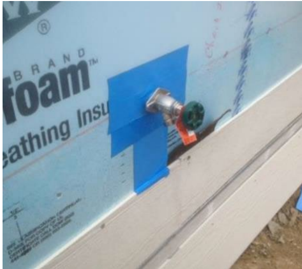
Figure 10-14. Place Butyl Adhesive Tape Around Faucet
