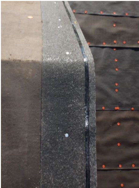
Figure 8-10. Starter Strip at Peak (Shown for 3-Tab)
