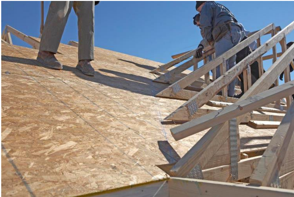
Figure 5-45. Progressively Smaller Tie-In Trusses
