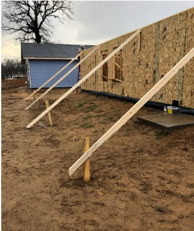
Figure 5-12. Ramps to Assist Loading Trusses
