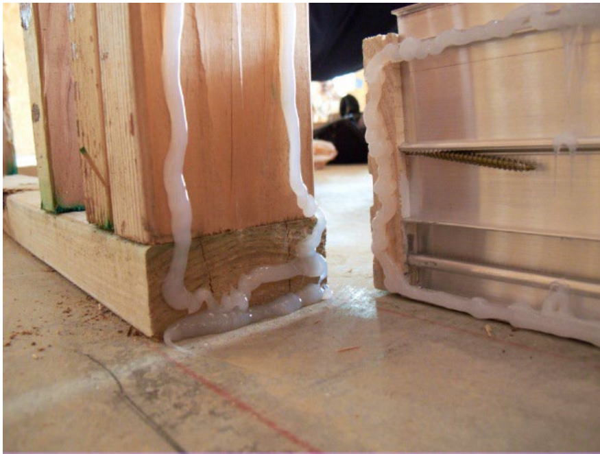
Figure 12-8. Apply Silicone Caulk to Jambs and Slab (Not the Threshold as Shown)
