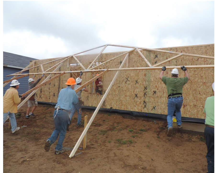
Step 4: As the top of the truss reaches the top of the wall, guide the truss along the wall for the volunteers
