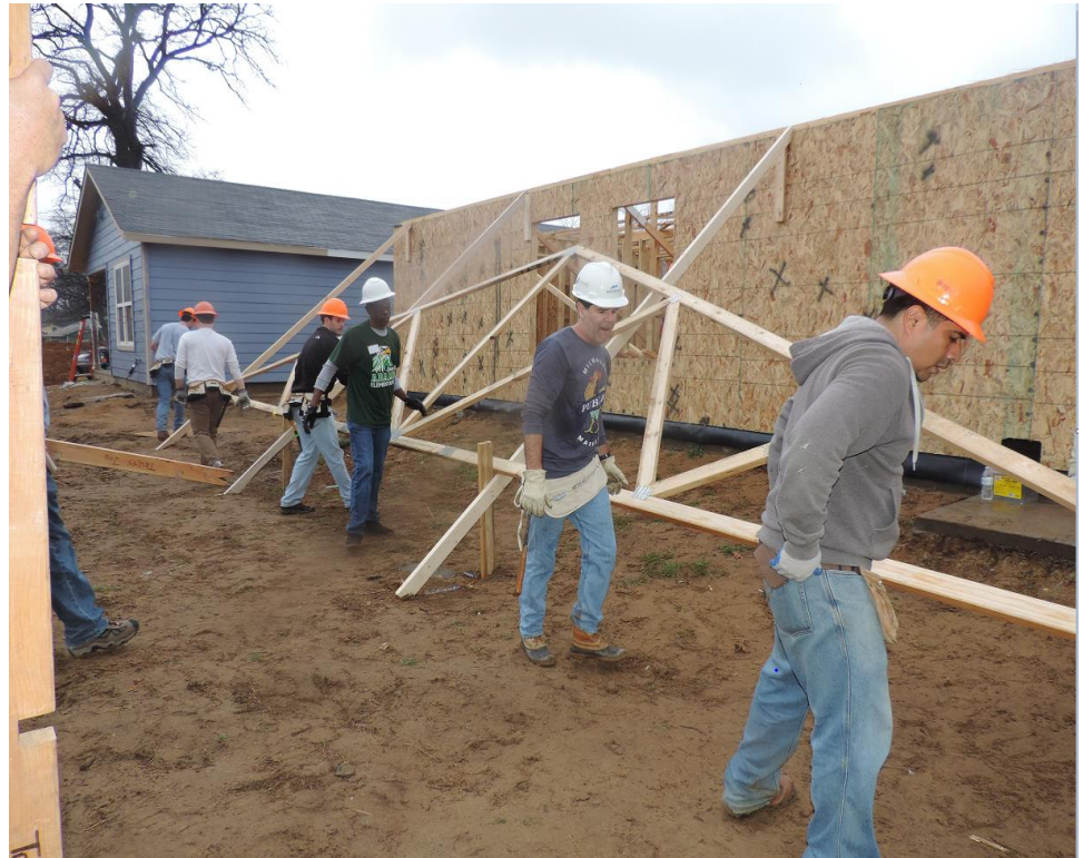
Step 2: Lay the truss on the bracing rails with the bottom cord resting in the "V" of the stakes
