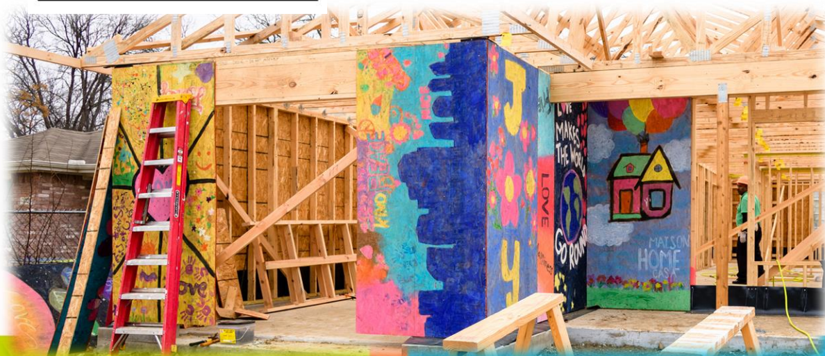
Figure 6-1. Use Full Sheets of Sheathing at Corners
