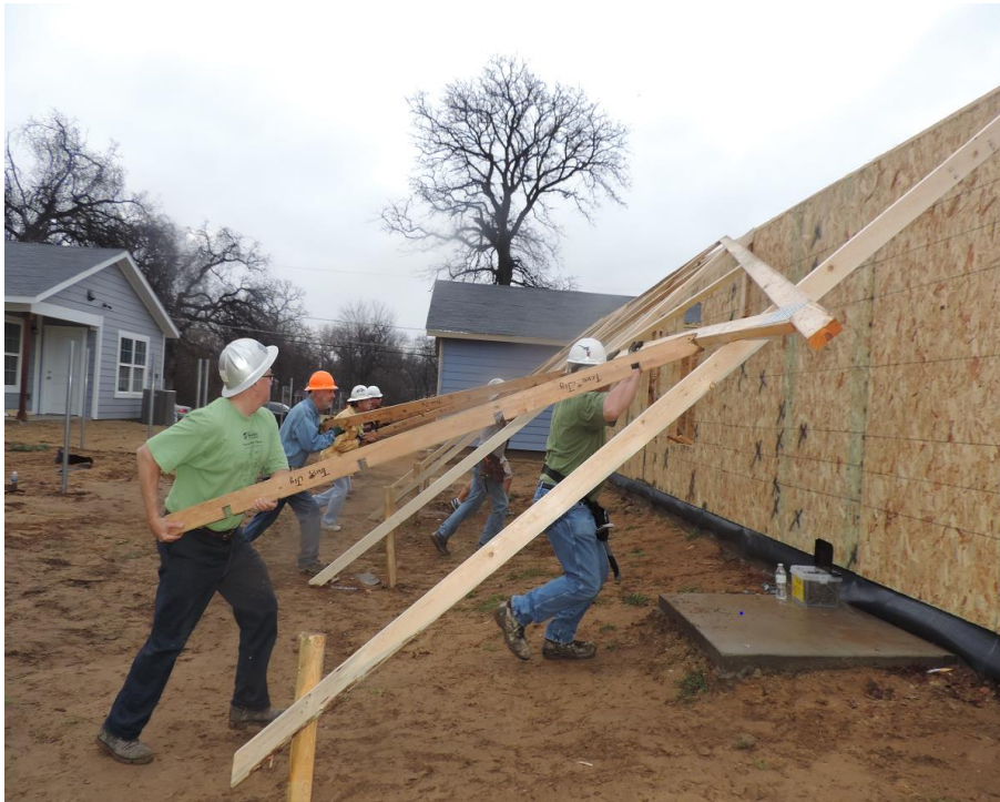
Step 3: Using push sticks, push the trusses up the bracing
