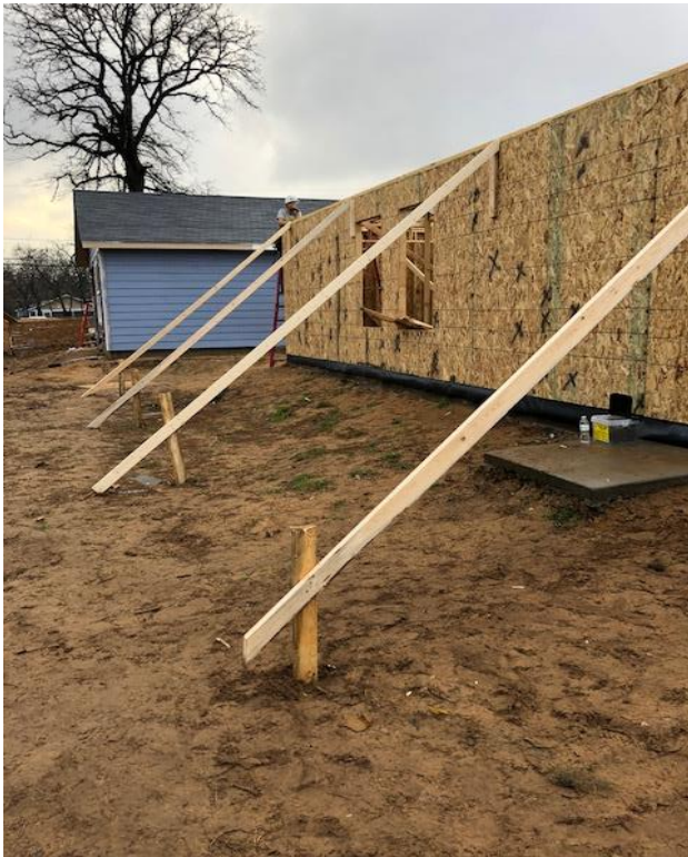
Step 1: Prepare the bracing to hold the trusses.
